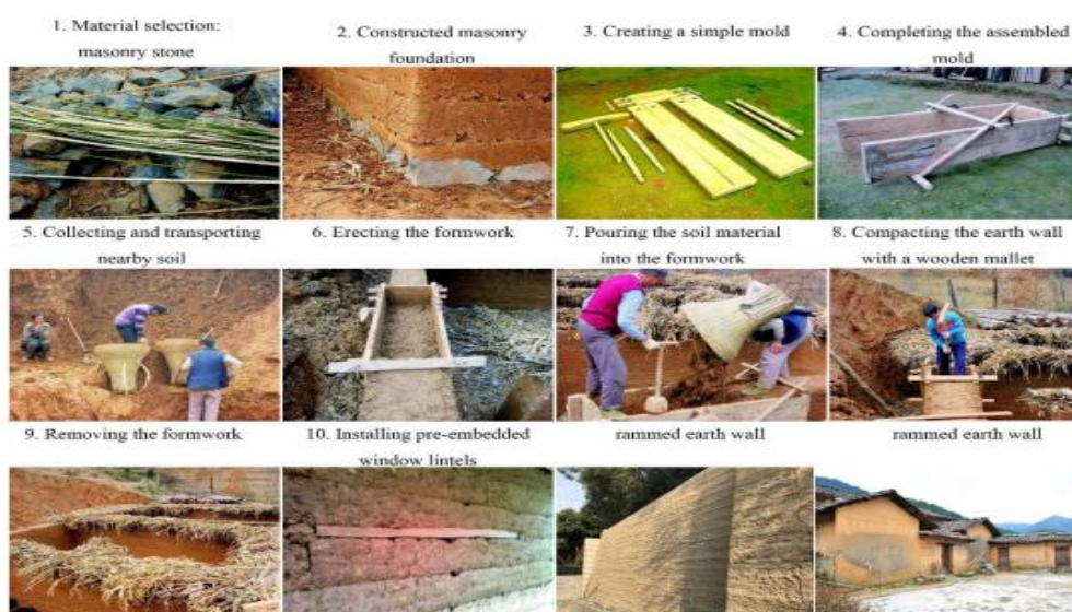
Figure 4: Construction process of rammed earth walls: site selection and material preparation; building the foundation, making molds; compacting the soil; layered compacting; smoothing the wall surface. During the construction process, it is necessary to consider drainage and moisture prevention measures for the walls, as well as insulation and soundproofing treatments. Safety should also be ensured.
