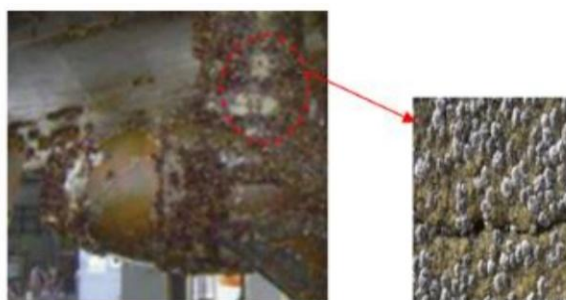
Fig. 11: Plate from an industrial seawater filtration device showing advanced paint degradation and replacement by biofouling organisms [37].
